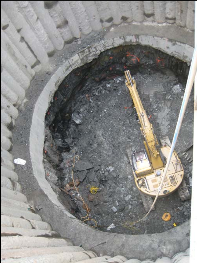
Shaft A – TBM Assembly Cavern
